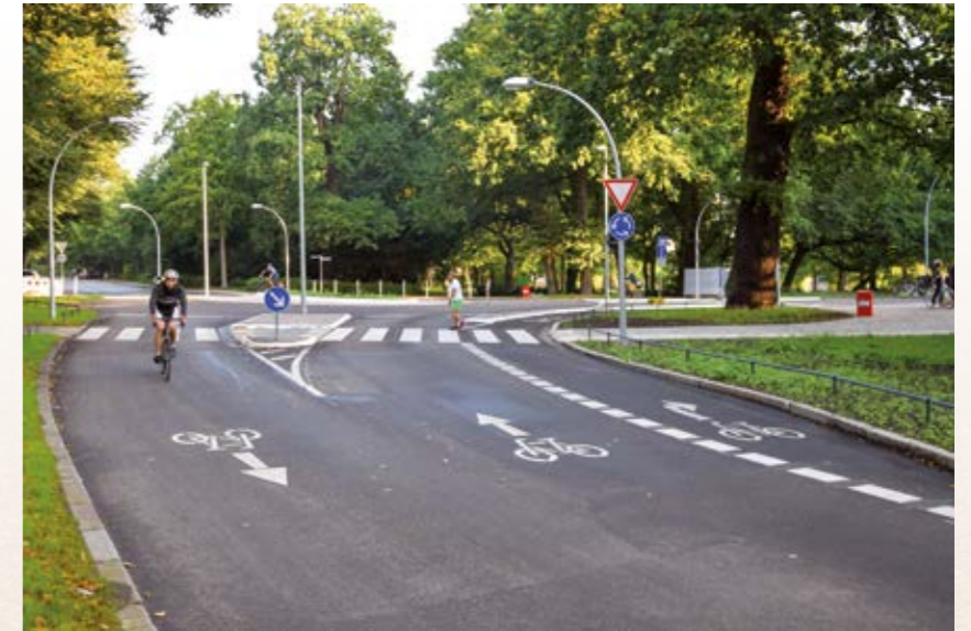
Completed bicycle path with separate turning lane.
