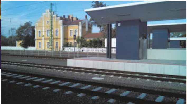
Island platform between two tracks in Törökszentmiklós.
